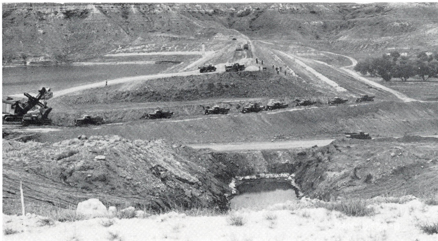
This photo, taken in the 30's, shows the construction of the dam and spillway. It was the largest dam in Kansas at this time.
