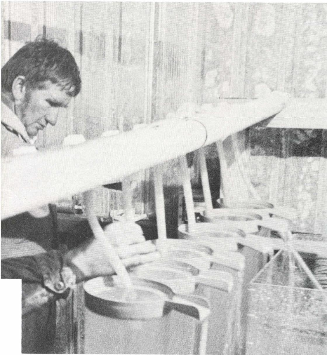
A small part of the plumbing at the Wilson striper hatchery. It's a complicated system with large storage tanks where water temperature can be adjusted and the water can be treated to kill fungi that attack eggs and fry. Biologists and technicians work day and night in shifts during the three-week spring hatching effort.
