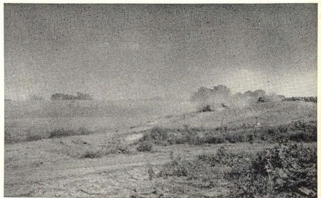
Men and machines are busily engaged in construction of the dam and spillway for the Montgomery County State Lake, being built on Coal creek, four miles southeast of Independence. Shown above are the large earth-moving machines that were used in the spillway work. The dam and control structure can be seen at left. The picture was taken from what will be the bottom of the lake.
