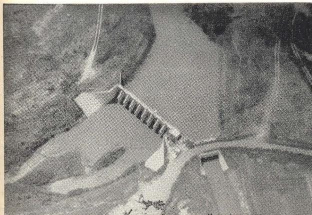
An aerial view of the diversion dam in Wet Walnut creek in Barton county. Flood waters may be seen being diverted through the control structure at the right into the inlet canal, thence on down into the Cheyenne Bottoms proper.—Photo courtesy Sharon Foster.
