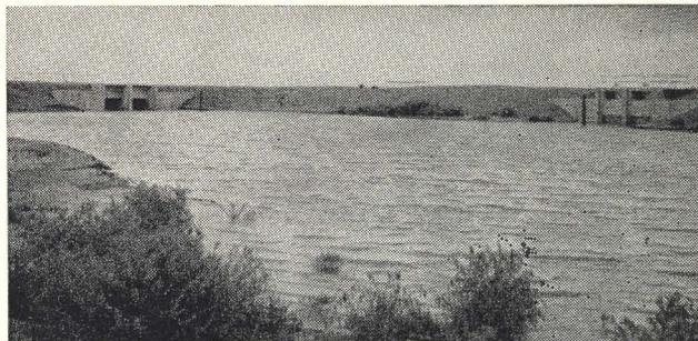
A view of the dikes and control structures in the Cheyenne Bottoms. The water, flowing into the area via the Wet Walnut inlet canal, is diverted through the control structure at the left into the main pool, where it will be impounded and used to flood the perimeter pools.
