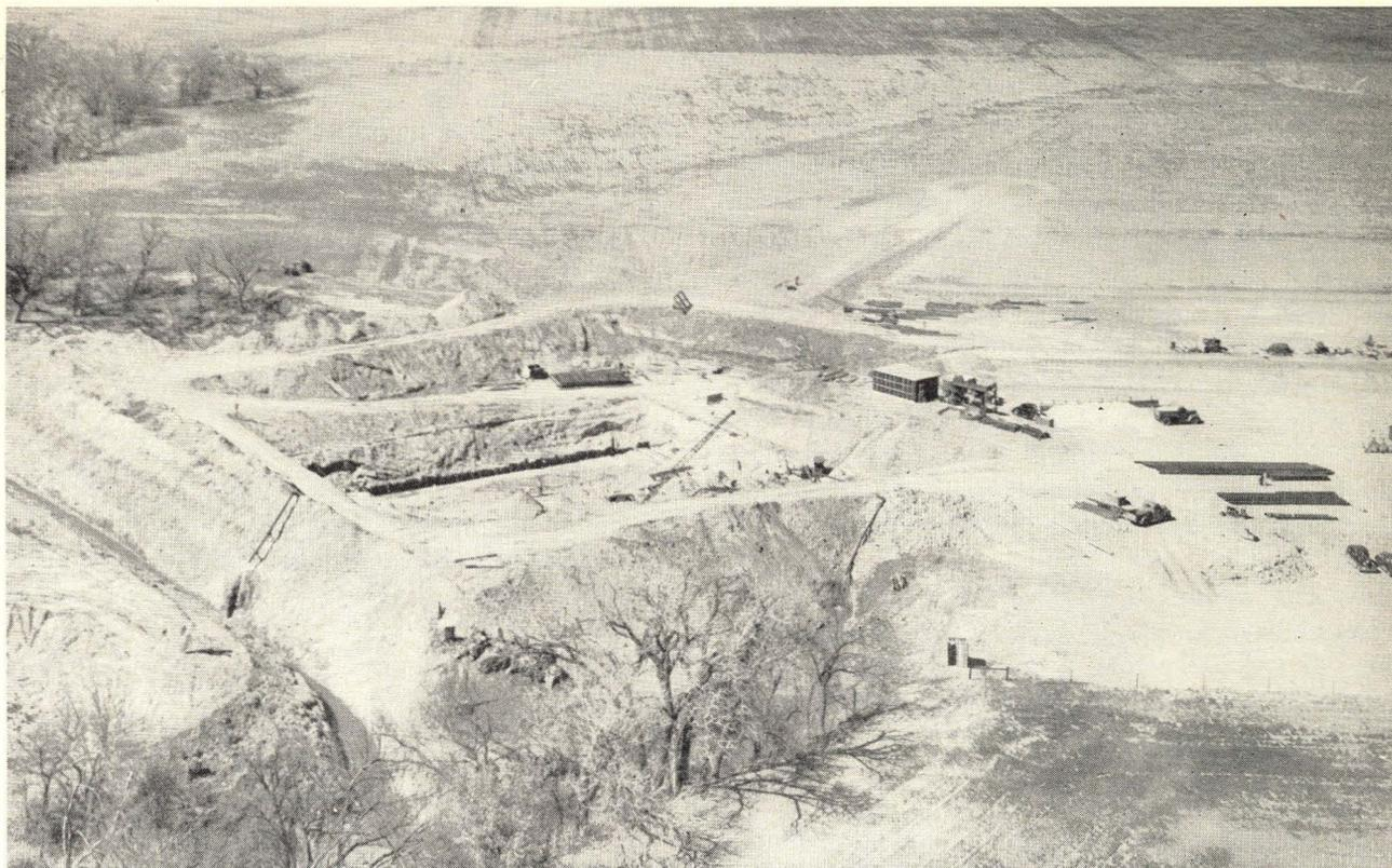
An aerial view of the diversion dam being built on Wet Walnut creek. The diamond-shaped earthen structure surrounds the site for the dam and blocks off Wet Walnut creek, which can be seen skirting the lower left-hand corner of the earthworks via a diversion ditch.
