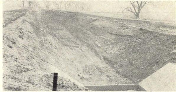
A mile west of where the diversion canal enters the Bottoms, a "drop-structure" has been built. This device, whereby the water drops twenty feet, will slow down erosion and scouring. The water falls into a "stilling basin," or "energy dissipator," that permits it to flow on into the Bottoms at a leisurely pace. The above picture shows the downstream side of the drop structure.
