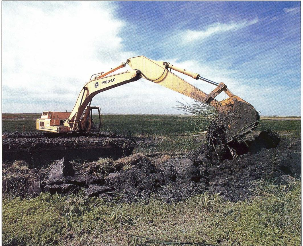
The backhoe has been used to remove silt and cattails, creating deep-water areas which are easier to keep cattail free. The silt is then used to build nesting and hunting blind islands.
