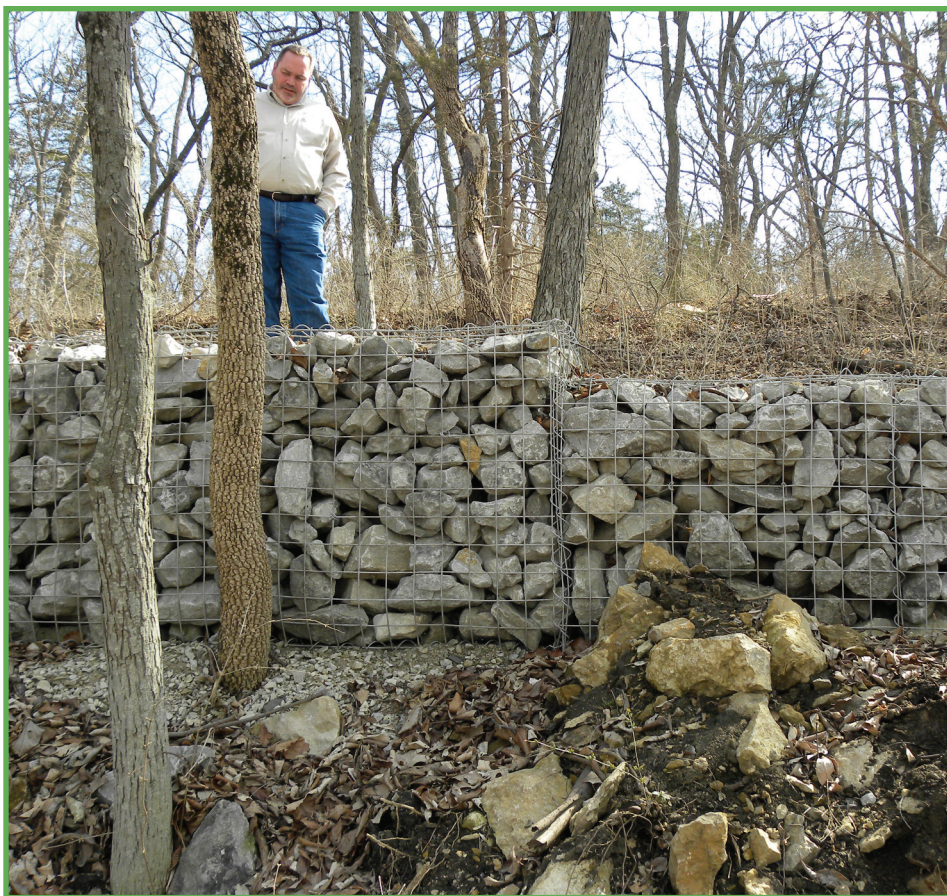
Gabion walls buttress trails across steep grades, preventing erosion and providing access for all — even emergency vehicles. Manager Jeff Bender examines his crew's handiwork.
