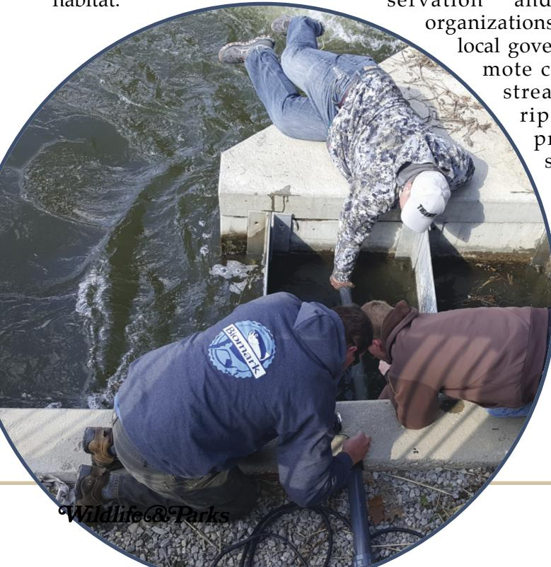
KDWPT stream biologists, Jeff Conley and Ryan Waters, install an antenna used to monitor fish movement in the fishway with the help of Peter Mackinnon, a post graduate researcher at Utah State University and technical expert in fish tagging. Jessica Mounts photo.
